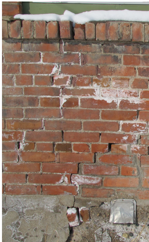
Fig. 15— Soiling and efflorescence at The Stoop, Rouleau
