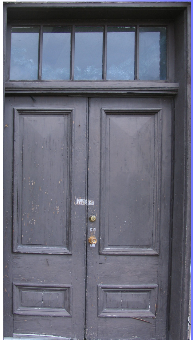
Fig. 14 — Raised-panel timber-frame doors with multi-light transom, McNaughton Stores building (1890) (Photo: M. G. Miller, 2011)
