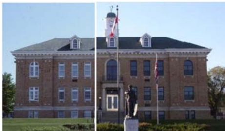
The Prince Albert Court House with the original white-framed wood windows (left) and the replacement black aluminum sealed units (right). Neither the colour nor the new window design replicates the original, thereby giving the building a very sombre appearance.
